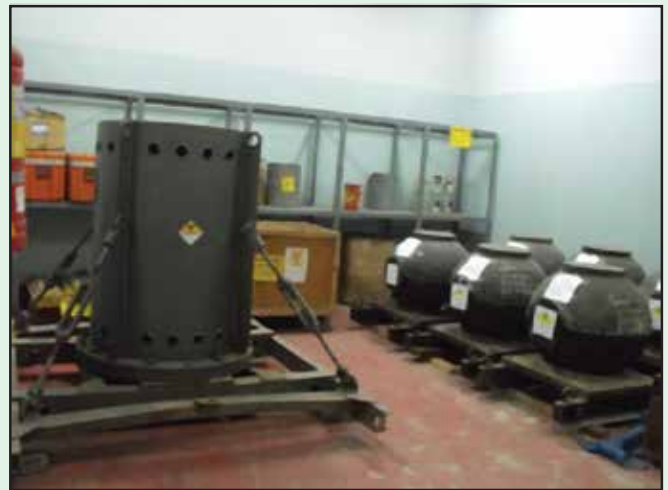
Storage of Disused Sealed Radioactive Source at CWPSF
